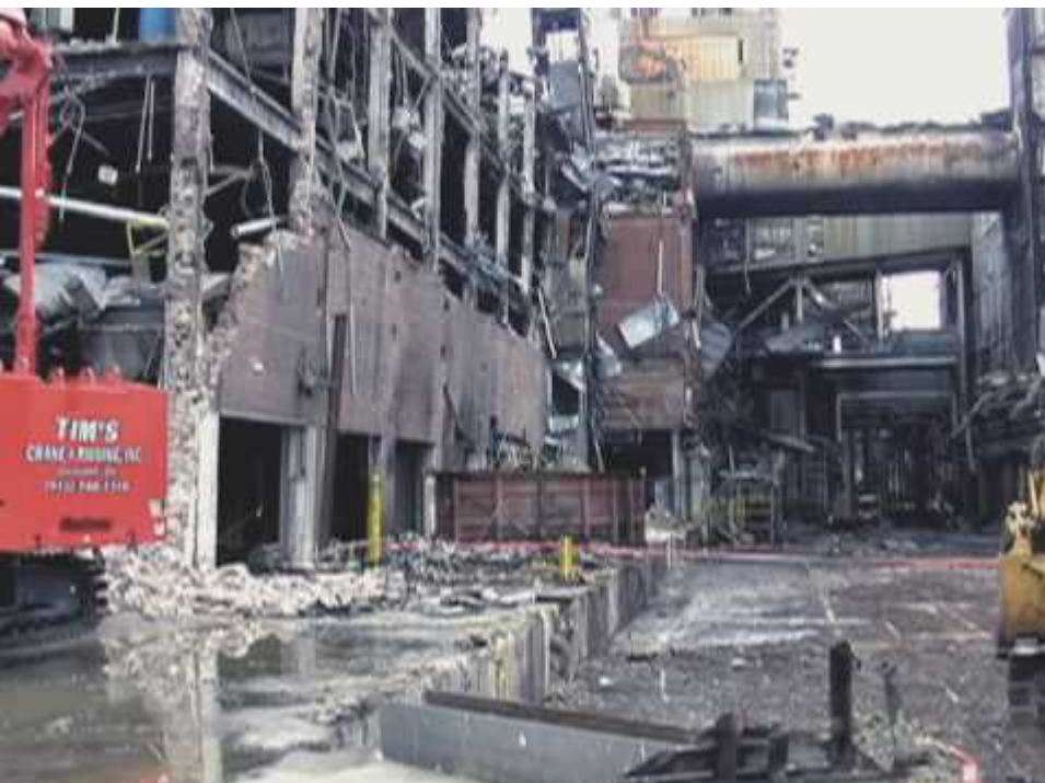
The Imperial Sugar refinery at Port Wentworth, Georgia, was destroyed by an explosion of accumulated sugar dust.
